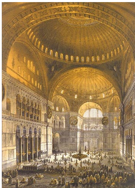
Figura 13. G. Fossati, Vista general de la nave central de Santa Sofía (1852), Victoria and Albert Museum.
