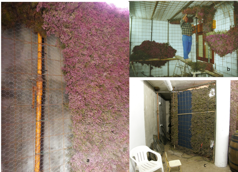
Figure 6. Assembly process of traditional Forest Crosses ( Cruces de Monte ) and Heather Crosses ( Cruces de Brezo ). a, initial construction phase showing the wire mesh framework for heather integration; b, structural details of a Municipal Cross (May 2001) during early heather insertion, featuring primary struts and mesh, with project supervisor Benito Laguna Albalade; c, composite view of a Mixed Cross (Democratic Union of Pensioners' Cross, May 2009) revealing internal components: iron reinforcements, wire mesh, cabling, and non-native slate fragments. Photos: A. Verde (a), F. Zamora (b, c).
