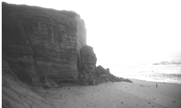
Fig. 10.- Part of the debris produced by the November 2000 rockfall. Photo taken in December 2000.
