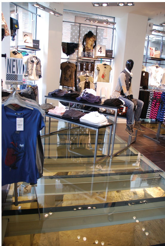
Figure 8. Wall from the 11 th century with subsequent modifications. It is visibly preserved underneath see-through glass. Shana shop, Granada. Lara Delgado Anés.
