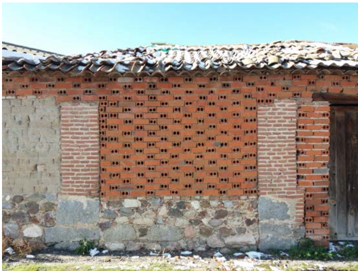
Fig. 6. Part of a construction in Santo Domingo de las Posadas (Ávila, Spain) built using various materials of industrial and pre-industrial origin. Photographed by the author.
