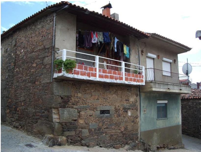
Fig. 7. House alteration involving the addition of a balcony in Poiares (Portugal). Photographed by the author.
