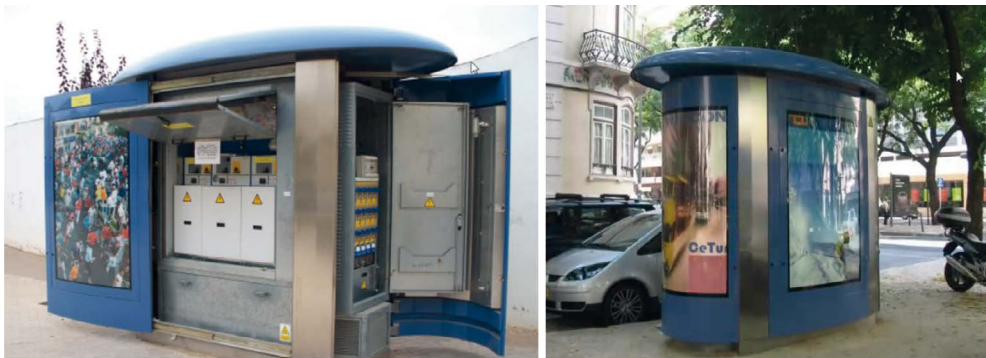
Figure 2. Out-of-home advertising incorporated into urban electrical substations through its innovative cover designed by TWELCON. [Source: www.twelcon.com ]
