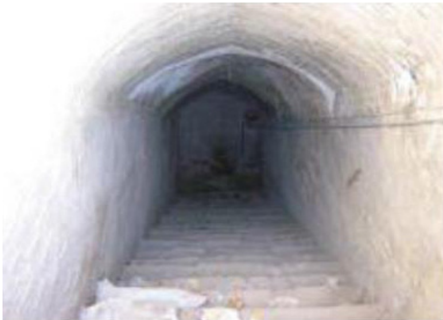
Figure 5. The location of the Pāshīr (the place under the ground where the water used to be taken from it) and staircase of the cistern in Darb Rīg of Arān and Bīdgul, Kāshān.
