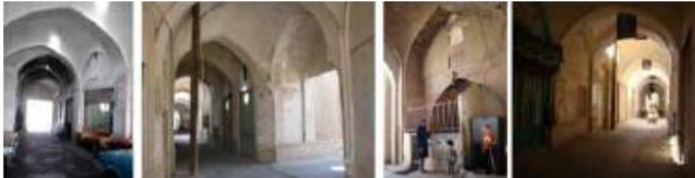
Figure 1. The great ability of Sābāt for (creating shade and natural ventilation) for long inhabitancy in Kāshān.
