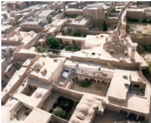
Figure 15. An image of the sunken garden of the soil architecture in the ancient constructions of Kāshān, Source [17].
